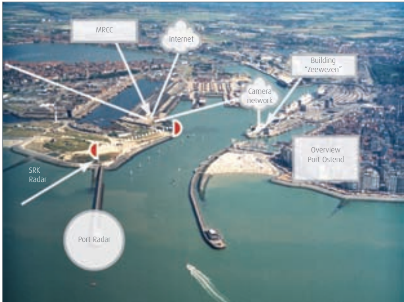
Outside view, multisensor inputs for MRCC
