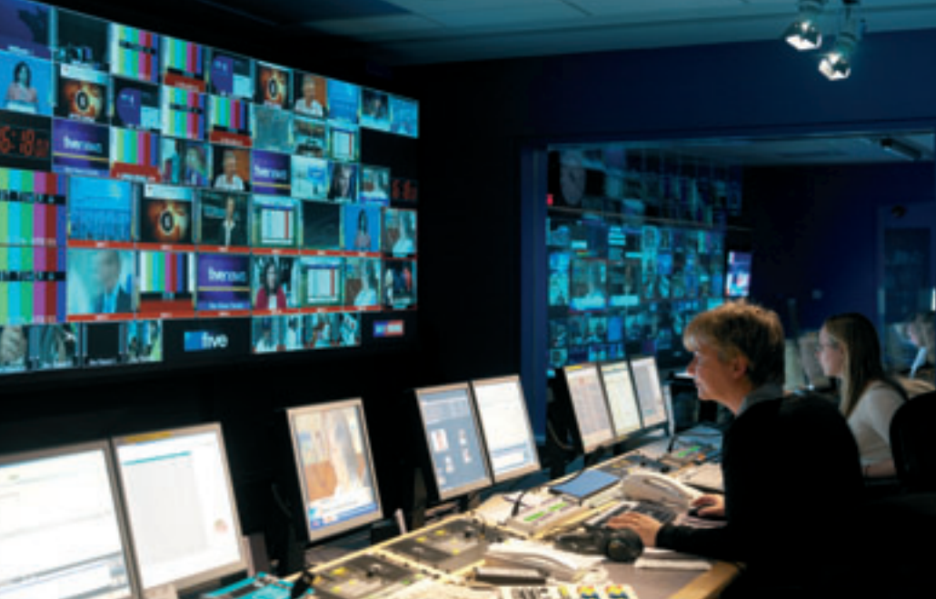
Left - Ingest/Playout Room equipped with a 3x1 67" rear projection display wall
