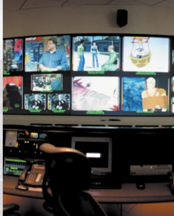
The outgoing TOC is used to monitor all outgoing feeds and return confidence feeds. It utilizes 3 OverView cPR84 display units incorporating 3-panel 1280x1024 pixel LCD technology with 3 HYDRA controllers.
