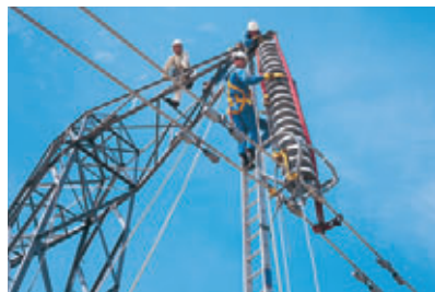
Utilities and process control centers
